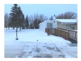
The outdoor shelters are refurbished shipping containers, each measuring 8' wide by 40' long, that are attached to the care homes. While there is no plumbing, they are fully insulated, air -conditioned and heated. But their most important feature is the ability for residents to visit others safely.
